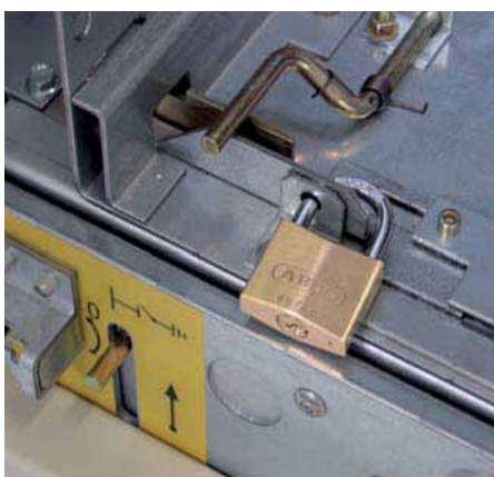
Fig. 10.13 Interlock of truck (optional)
