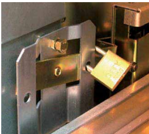
Fig. 10.12 Mechanical lock-out for shutter (same principle for left-hand and right-hand sides)
